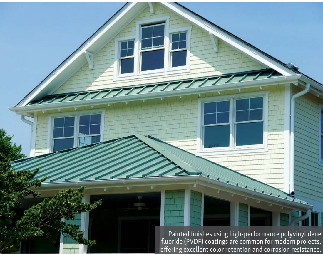
The bold ridges of batten seam metal roofing stand out as a distinctive feature of the building's design.
