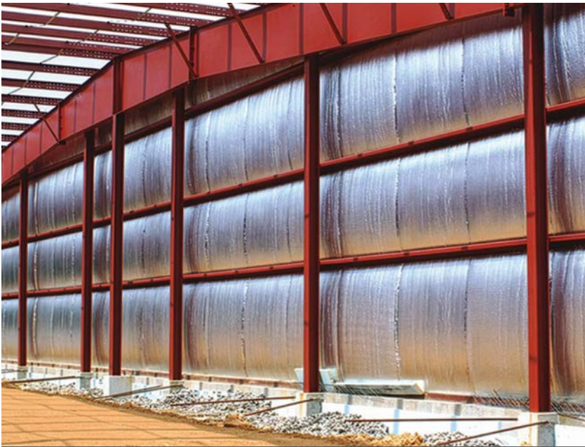
Reflective insulation is the most effective defense against radiant heat gain and loss in metal buildings.
