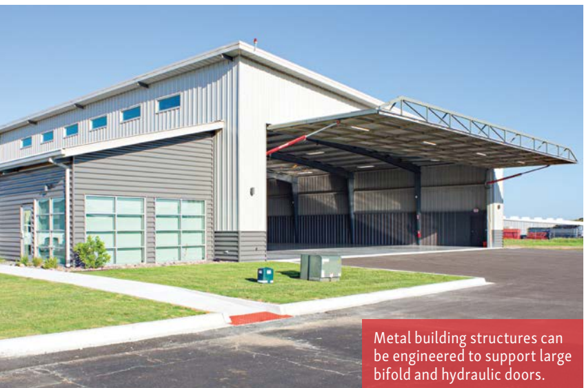
Using bifold doors on a metal building allows for the design of large doors.
