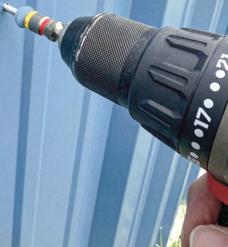
The fastener washer forms the primary seal in an exposed-fastener roof system.
