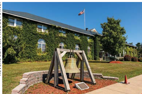
Revere Copper Products' campus in Rome, N.Y.
