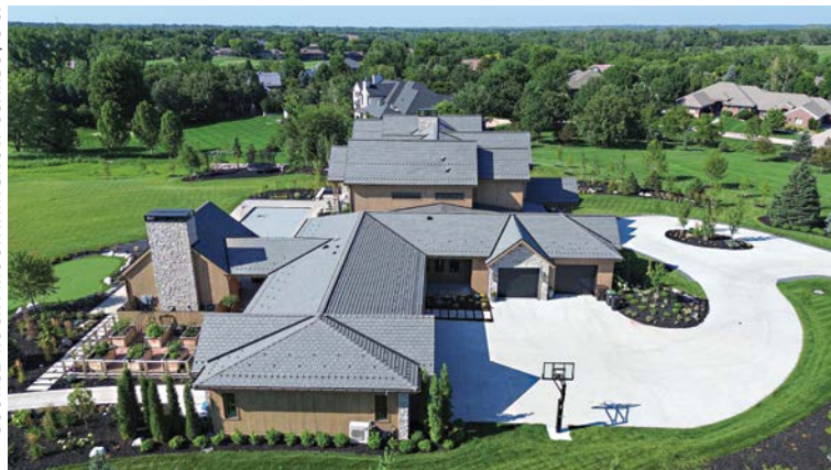
Winning project in Lincoln, Neb., by White Castle Roofing.
